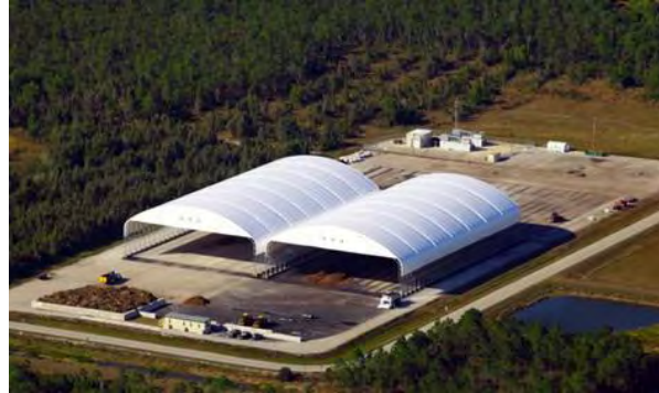
Through a public/private partnership, Synagro financed the compost facility with internal funds and initiated construction in September 2013; the facility was ready to begin accepting biosolids within five months.
