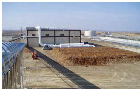
Synagro utilizes an enclosed biosolids receiving and mixing building along with biofiltration in its compost system that controls VOCs and odors for the surrounding area.
